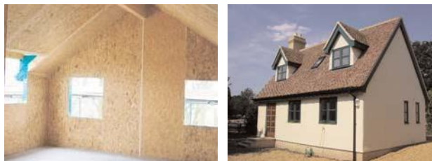
Typical interior after erection and house supplied by Edward Halford Ltd
