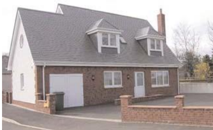
Traditional house supplied by SIPit (Scotland) Ltd
