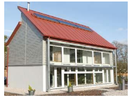
The BASF eco house built with SBS SIPs
