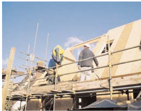
Erecting small house in Cambridgeshire (Edward Halford Ltd)
