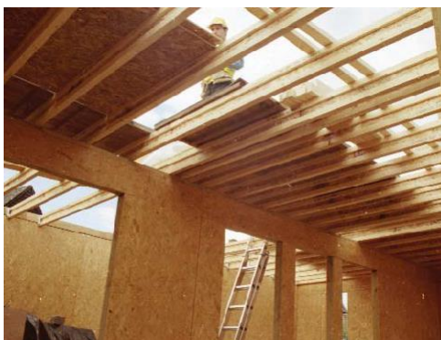
Engineered floor joists in SIP house
